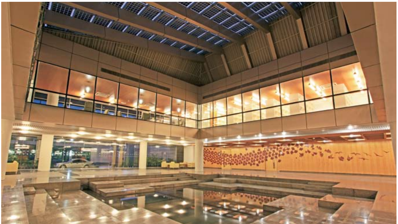
Solar photovoltaic panels form the roof of the atrium of the learning centre, generating green power.
