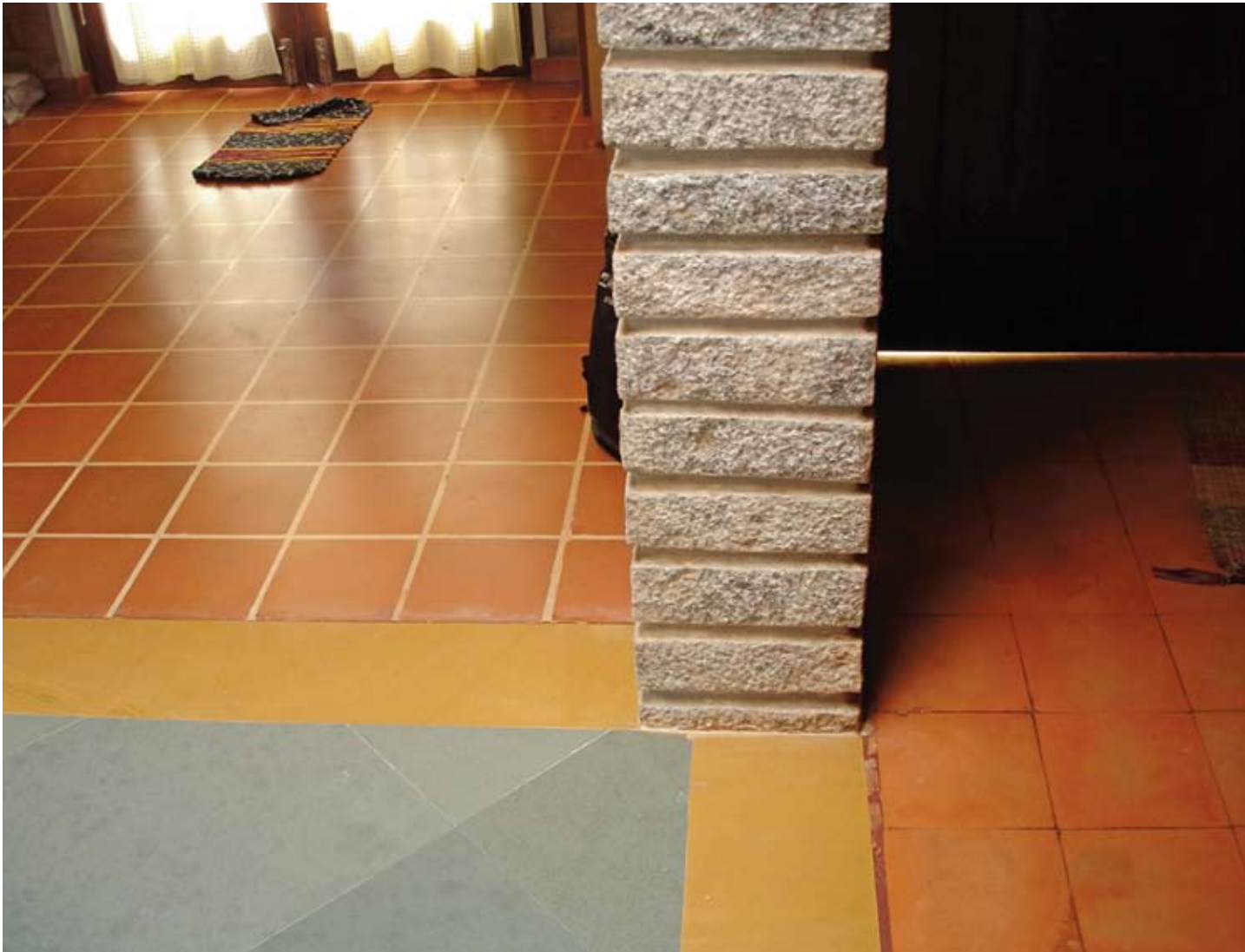
Clay tile flooring, Kanavi residence designed by Ar Deepak Godhi
