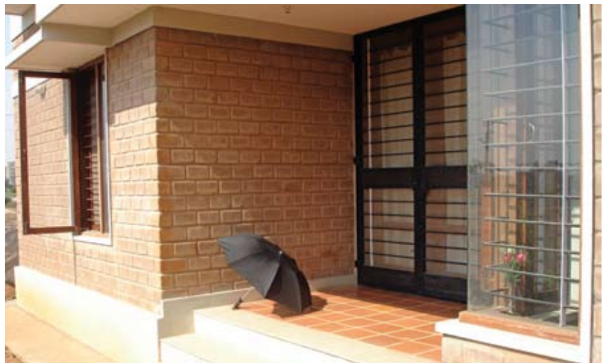
Mud Blocks, Less Plaster
