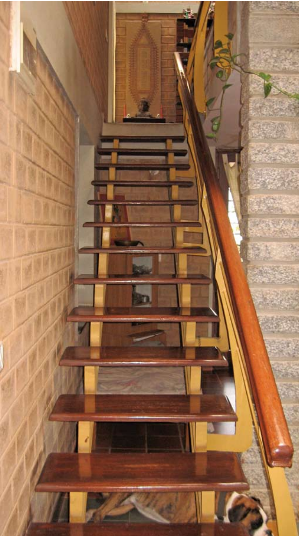
Wood and steel staircase
