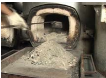
Figure 7. Incinerator and incineration ash (Photo Courtesy: Passco)
