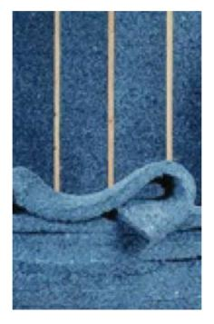
Polyurethane — Expanding spray-on polyurethane foams are quickly becoming very popular. They offer the highest insulation value for a given thickness and, because of their expansion during installation, are excellent at eliminating air leakage.
