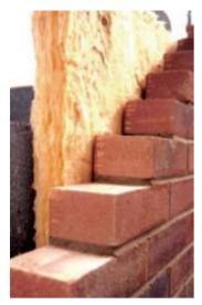
insulating a structure beyond building-code requirements is a fundamental principle of green building. Many green builders take advantage of the low cost and ease of installation to super insulate and save money that they can use for other green features.
